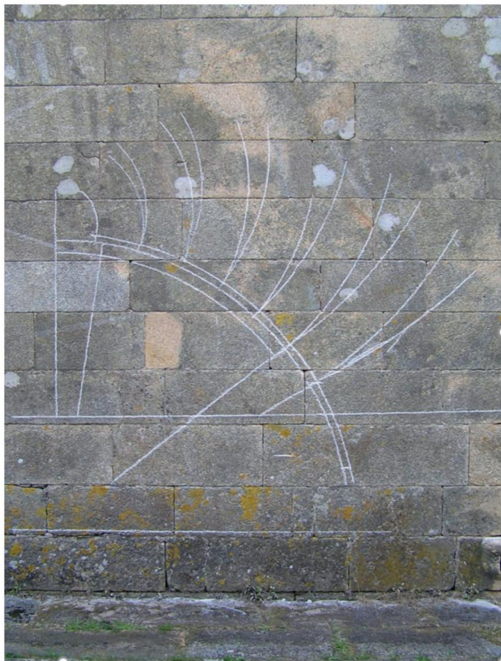
Carnota, parish church. Full-size tracing for a quarter of sphere vault. Photograph by Miguel Tain
