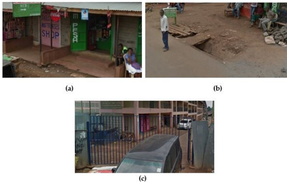
Figure 13. Hot-spot 1: territoriality elements. Porticos (a), drainage system (b), and fences (c) (source: Google maps street views).
