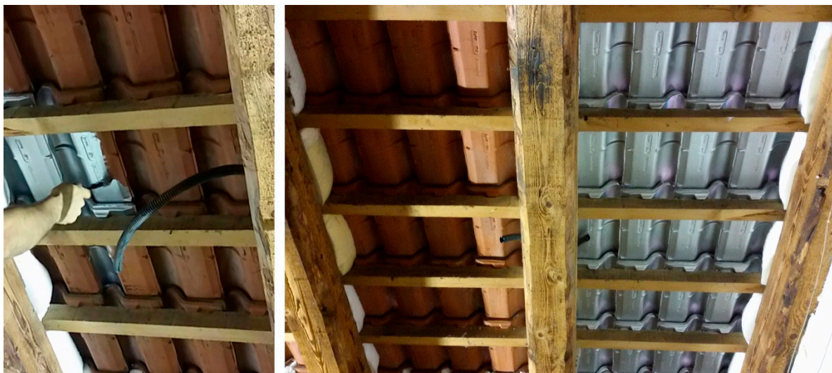
Figure 1. Application of an interior radiation control coatings (IRCC) in roof attic.
