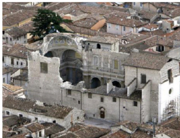
Fig. (3). Santa Maria church in Paganica (Italy) after the earthquake of 2009.
