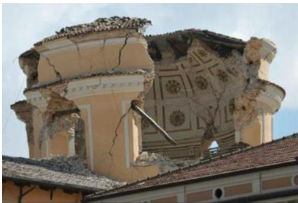
Fig. (2). Dome and drum of the Anime Sante Church in L'Aquila after the earthquake of 2009.
