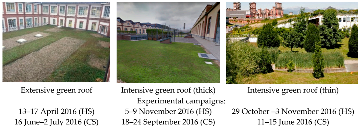
Figure 4. The extensive and intensive green roofs analyzed during the heating (HS) and cooling (CS) seasons.
