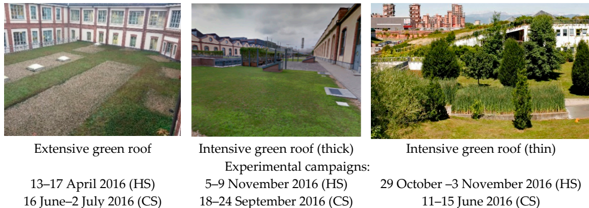
Figure 4. The extensive and intensive green roofs analyzed during the heating (HS) and cooling (CS) seasons.
