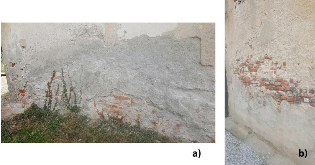
Fig. 1. Some examples of plaster detachment on historical walls due to: a) damp action from capillary rising, b) the action of freezing-thawing freeze-thaw cycles.
