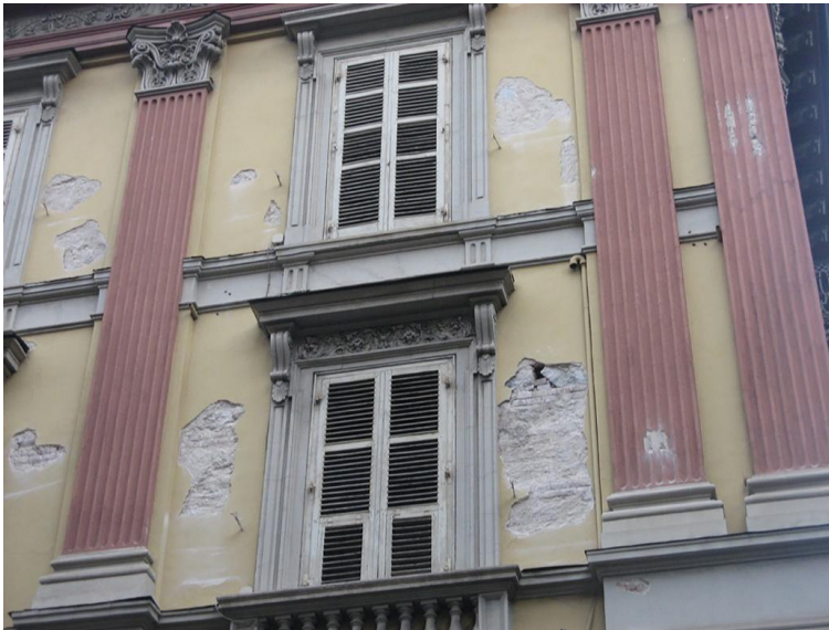
Fig. 2. Example of the mechanical incompatibility of patches made by cement mortar in a historical plaster based on lime mortar. The noticeable difference in stiffness of the concrete patch against the original lime-based plaster has favored the detachment under thermo-hygrometric stress.
