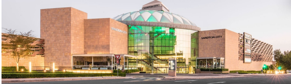
Figure 3 | Sandton City, the new Johannesburg Central Business District.
