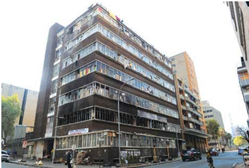
Figure 4 | Hijacked building in Johannesburg CBD.
