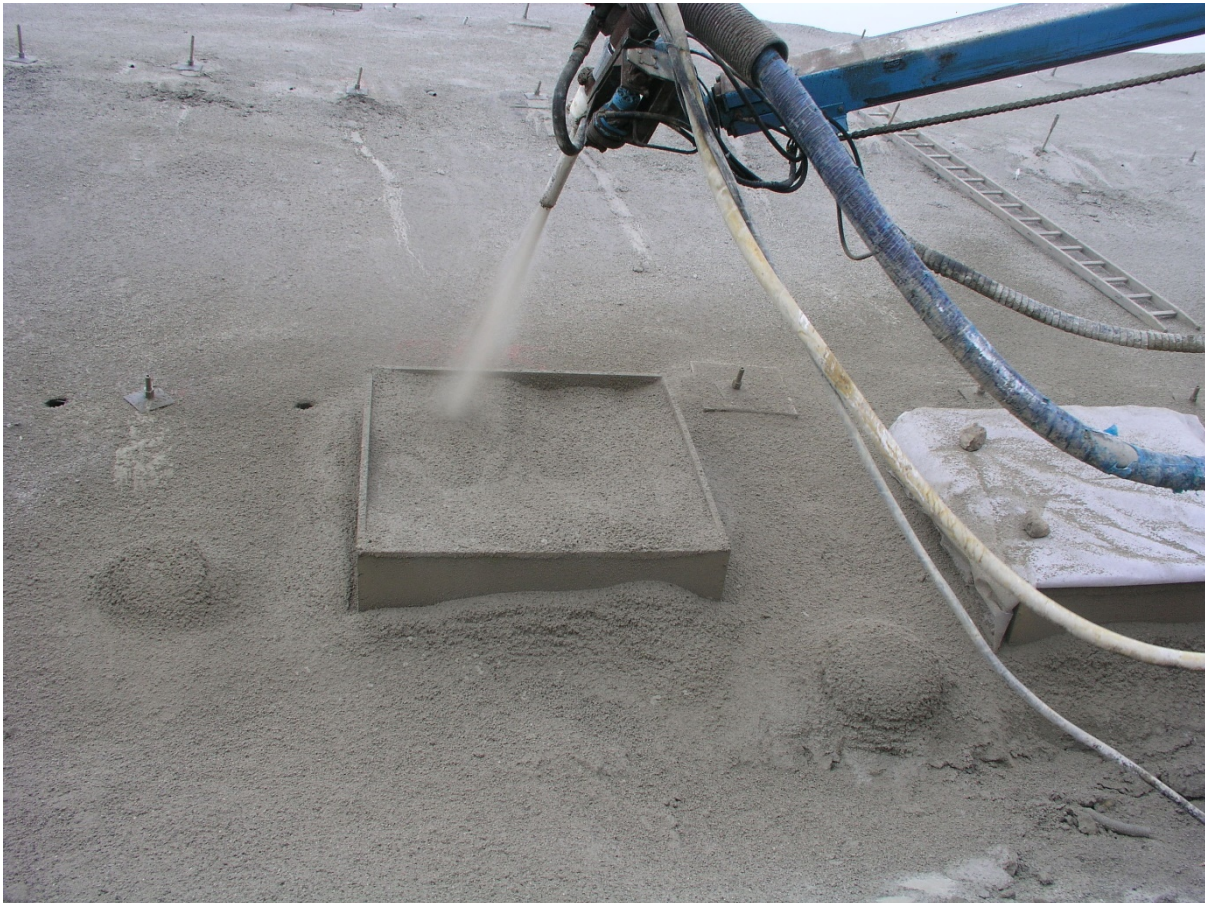
69 Fig. 1 Sprayed concrete trials in a job site.
