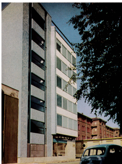
Figure 1. Domenico Morelli, SIP Office Building, Turin, 1951-57 (with T. Finzi; structure by A. Antoldi; construction company: Rain-eri). The face of the prism overlooking Via Promis is distinguished by the vertical stair block [2].
