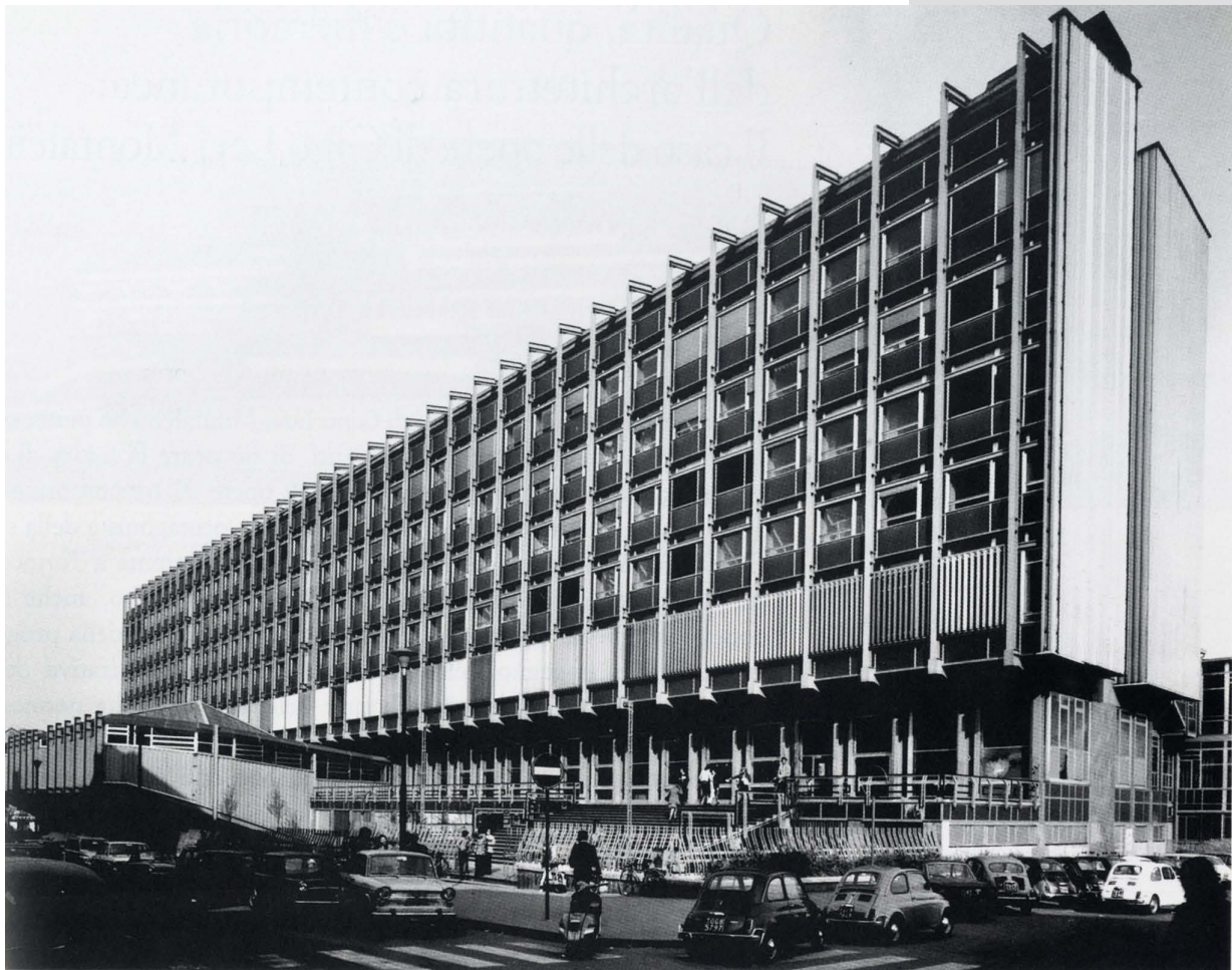
Figure 4. G. Levi Montalcini, D. Morelli, F. Bardelli, S. Hutter, Social Sciences building of the University of Turin (Palazzo Nuovo), Turin, 1961-68 (T. Finzi; structure by G. Donato).
