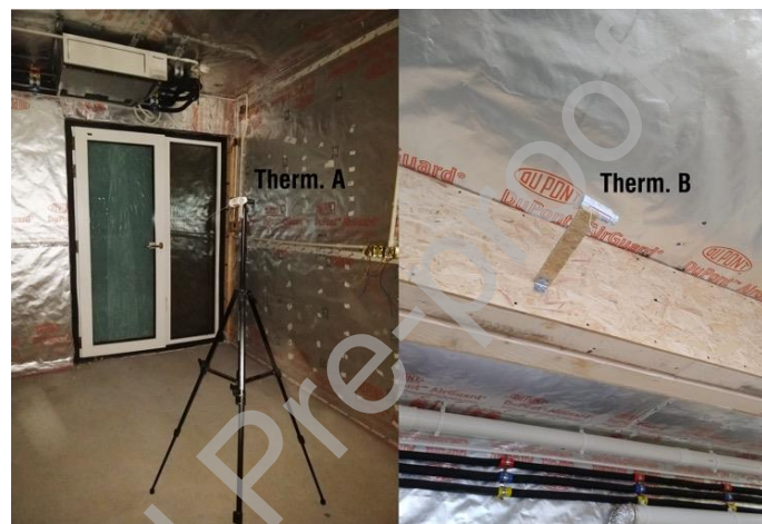
Figure 5: Picture of the placement of temperature sensors
