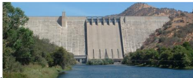
Figure 1: Downstream view of Pine Flat Dam
