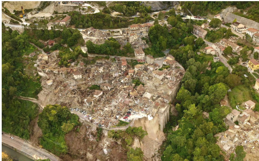
Figure 5. Model of Pescara del Tronto after the August 2016 Earthquake events.
