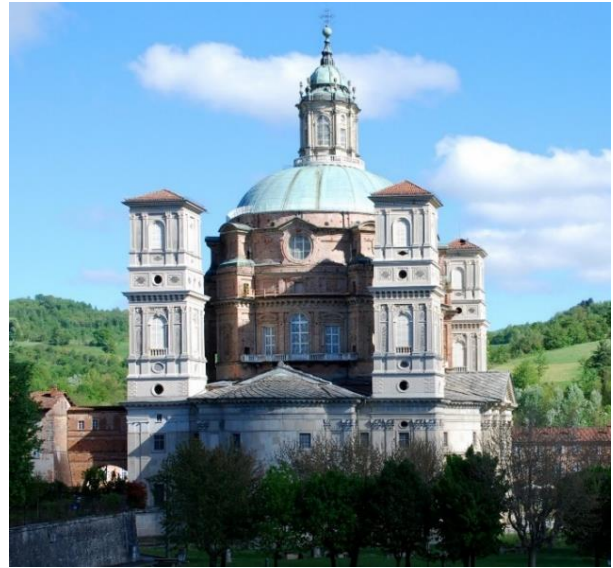
Figure 2. External view of the Sanctuary of Vicoforte.
