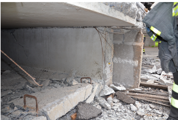
Figure 2: Collapsed joint.
