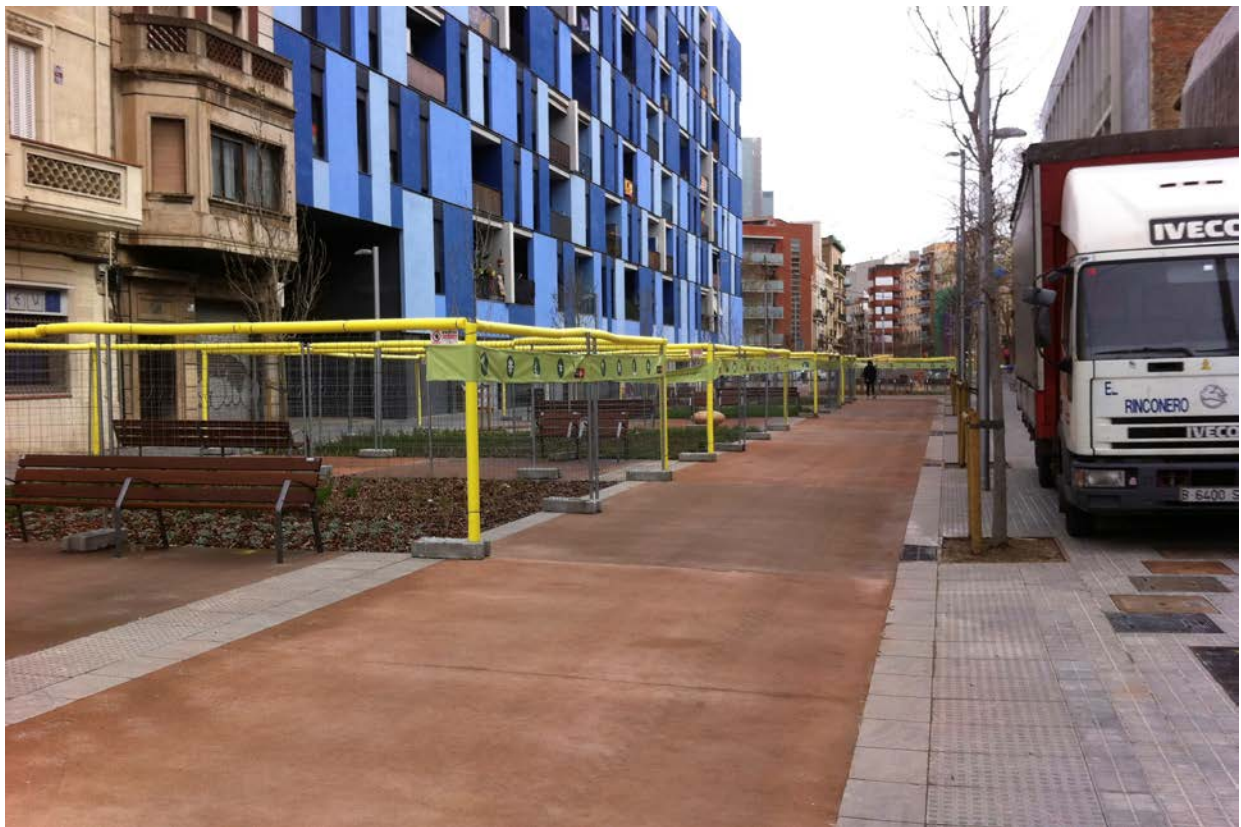
Figure 11. Structural implementation of the Poblenou SM: inner streets (2018). Source: authors
