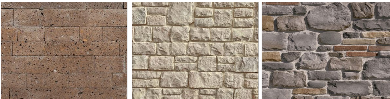
Fig. 6. Examples of Etruscan tuff masonry wall, limestone masonry wall and huddled/mixed stones wall.
