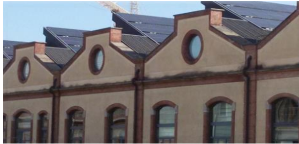
Fig. 1 View of the PV system under test
