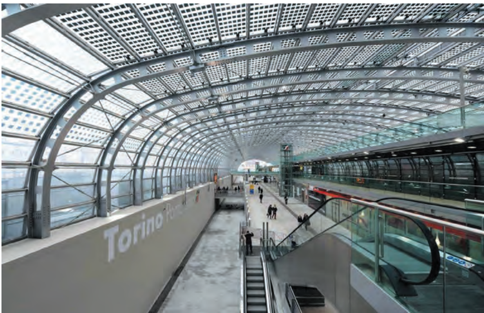
Figure 5: Torino Porta Susa, view of the ground level. ( Ansa/Di Marco )
