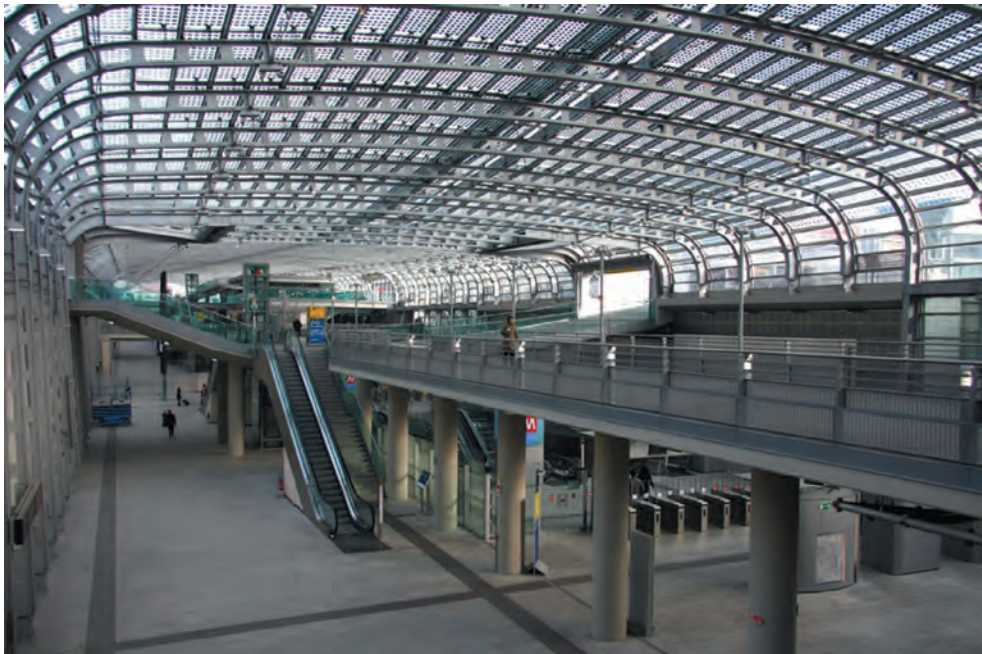
Figure 6: Torino Porta Susa, the connection between the ground floor and the entrance to the subway. ( www.fsnews.it )
