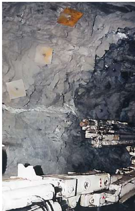
121 Figure 4. Very irregular profile after D&B tunnelling due to rock joint pattern and poor contouring techniques. 122 Suggested D = 0.8 . (Photo by C. Oggeri)
