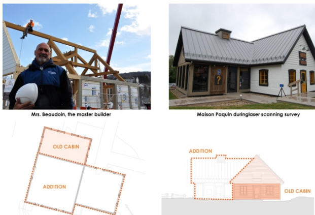
Figure 2. Maison Paquin restoration
