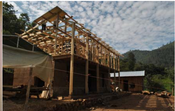
Fig. 8 - The modular wooden structure in Pensamiento.
