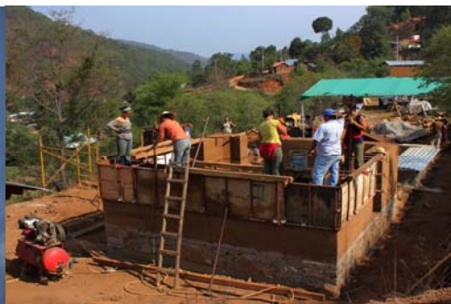
Fig. 10 - Mechanized process of compaction of rammed earth walls in Pensamiento Liberal.
