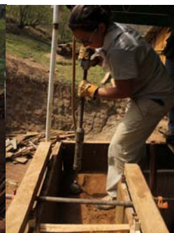
Fig. 11 - Compaction with pneumatic piston.
