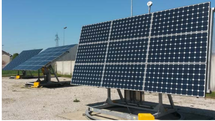
Figure 3. Example of misalignment between the plant A_{ts} (right-side of the picture) and the plants D_{ts} and E_{ts} (left-part of the picture).
