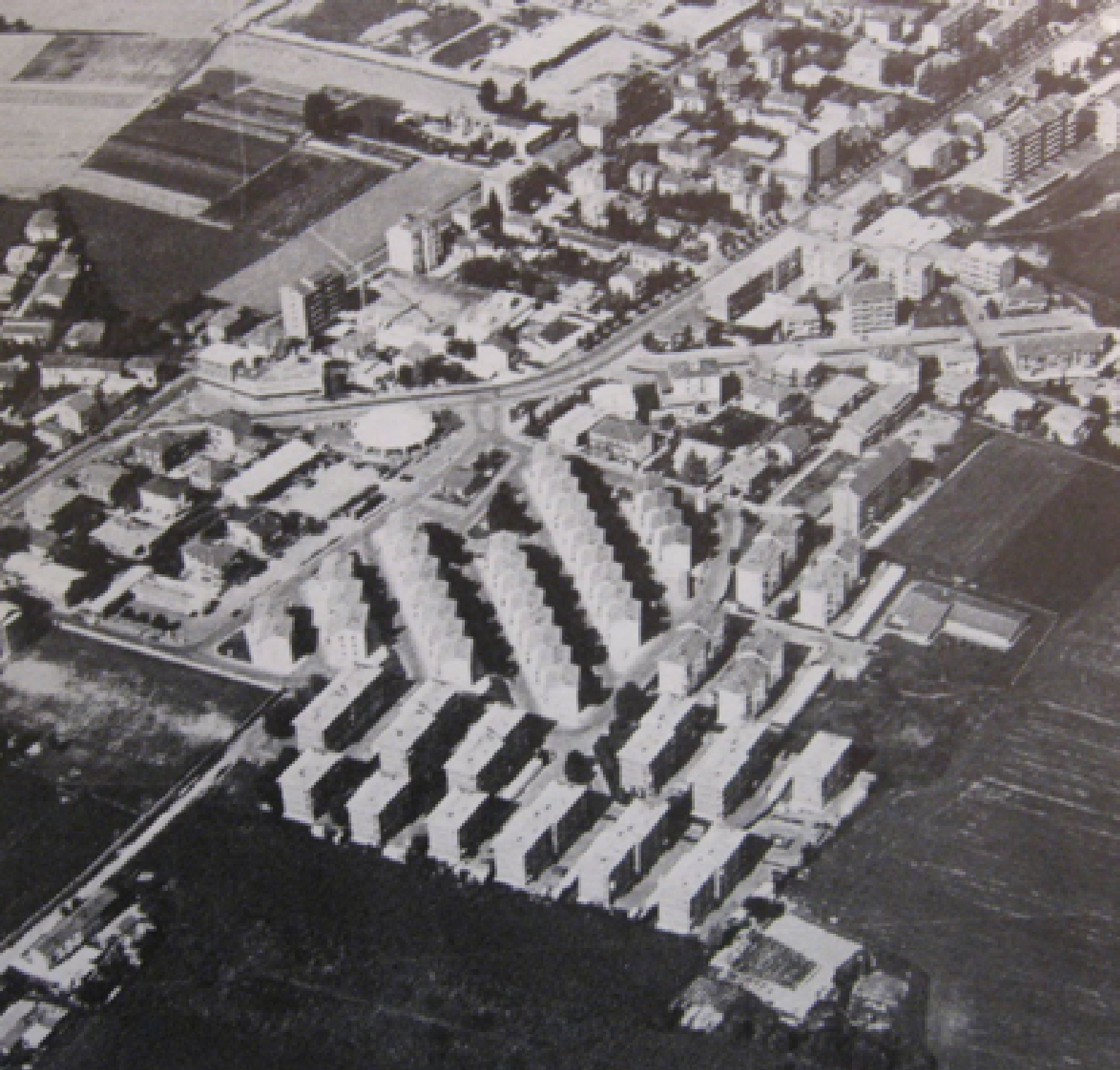
Alessandria, overview of the Cristo district with the social housing block built in the 50s and later (source: "80 anni di IACP nella provincia di Alessandria").
