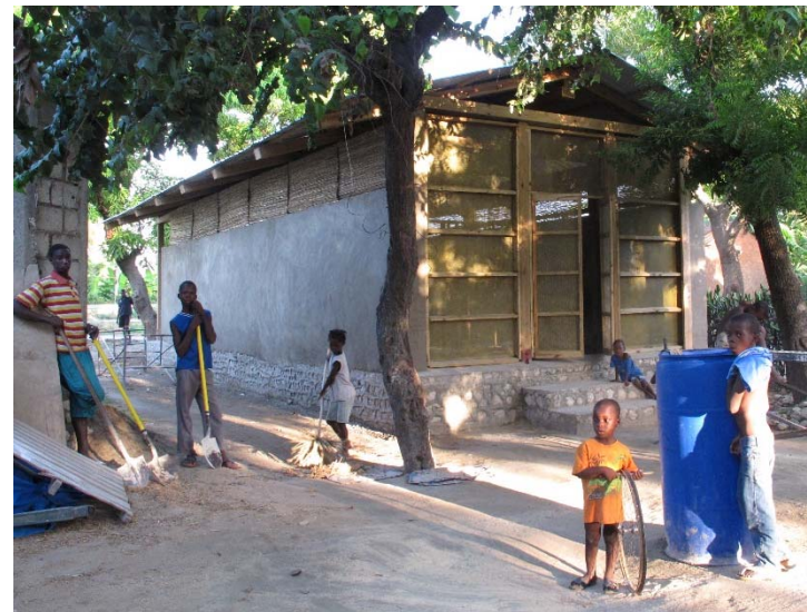
Fig. 16. A typical straw bale obtained by using the prototype press and the background the warehouse built by ASF in Haiti using the bales.
