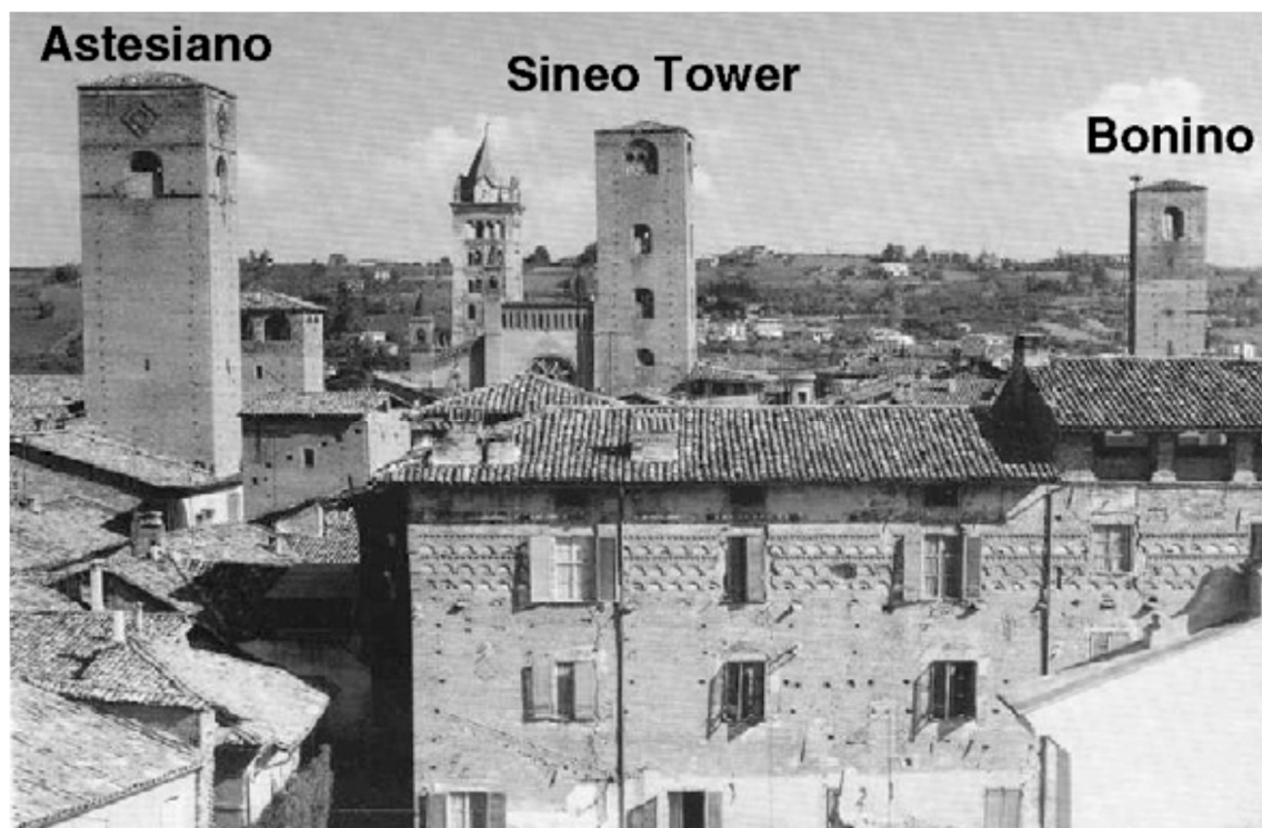
Figure 1. View of the Astesiano, Sineo and Bonino towers in Alba.
