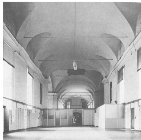
Figure 7. Hospital San Giovanni: photograph inside the vault.
