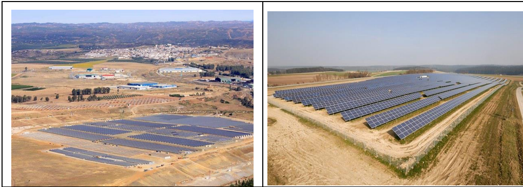
Fig. 3 (left) and 4 (right). Views of the PV plants of Seville and Herestried (Germany).
