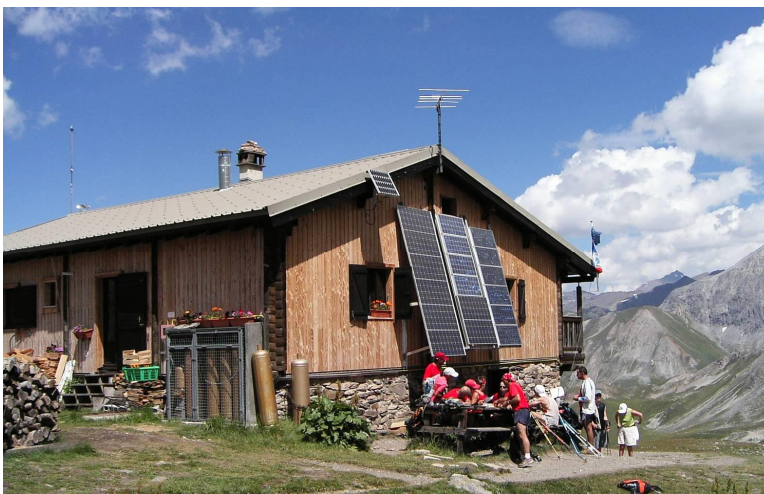
Fig. 9. Various forms and colors of a PV plant for an alpine shelter in Italy (Susa Valley).
