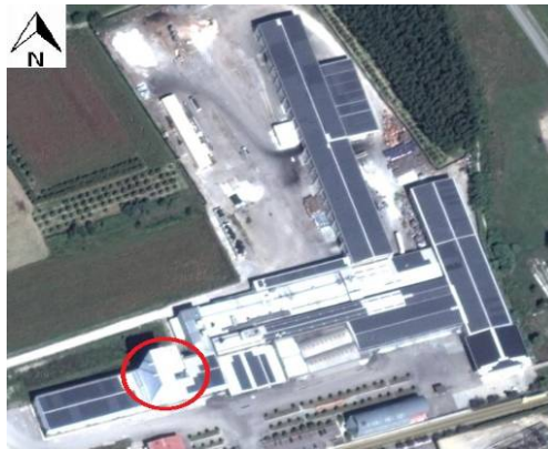
Fig. 2. Satellite image of the 2.5 MWp BIPV system.
