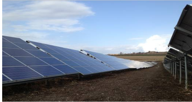
Fig. 1. Photo of two successive rows of PV modules in the GMPV system.
