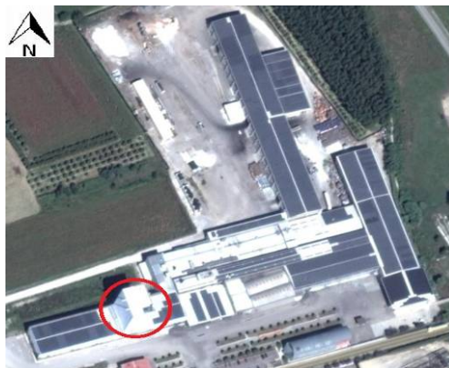
Fig. 2. Satellite image of the 2.5 MWp BIPV system.
