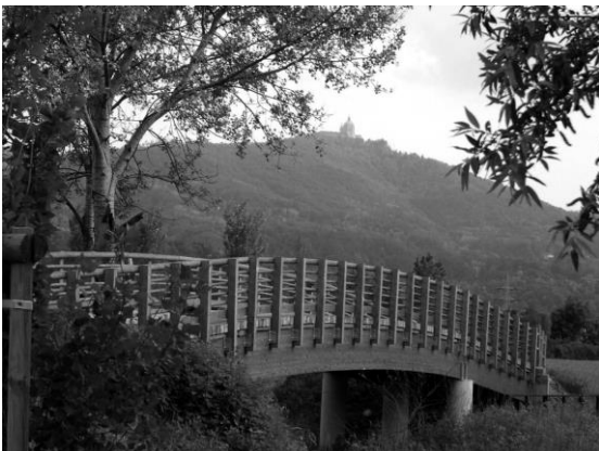
Figure 5. A new pedestrian bridge.
