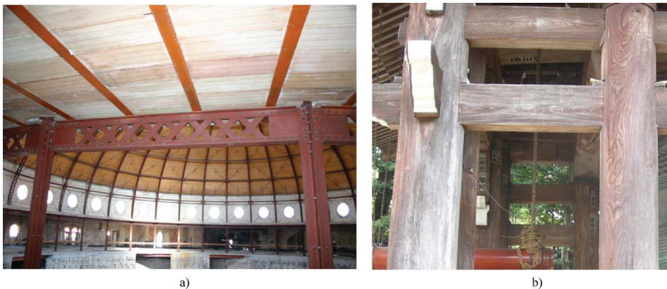
Figure 10. Photographs of the rigid steel frame solution (a), and timber solution adopted by a Japanese Torii (b).
