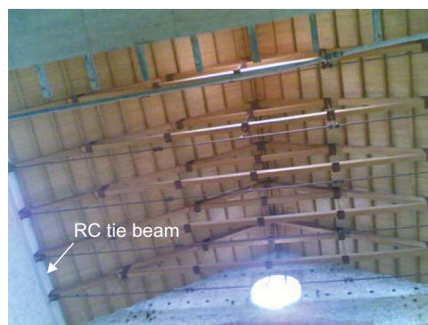
Figure 19. Photograph of the fly tower: particular of the reinforced concrete tie-beam.
