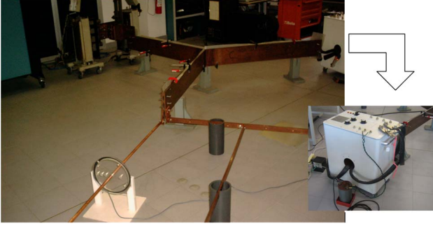
Fig. 7. Y-bar system, reference current transformer, and RC arrangement.
